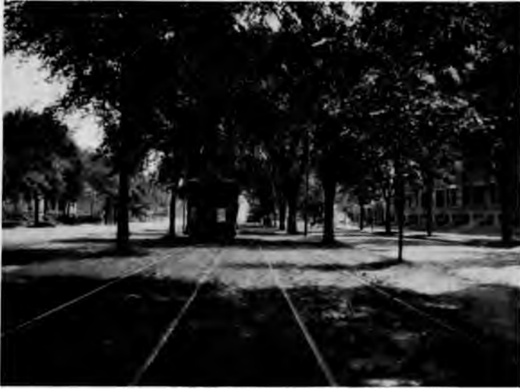
A thoroughfare, 175 feet wide, through a Boston suburb—A model for the treatment of University Avenue, Verona Road, Sun Prairie Road, and other outlying highways of Madison.
